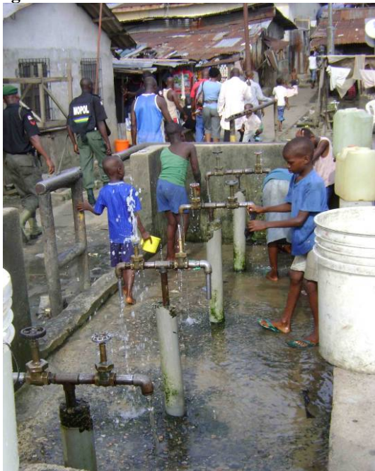
As part of its community development programme, Shell constructed a borehole in the community which serves as a major source of water supply. The borehole has been running without control because the handles have gone bad. © R. Precht
