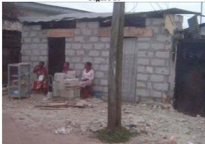
Three ladies in front of their partly-demolished eatery in GRA © R. Precht
