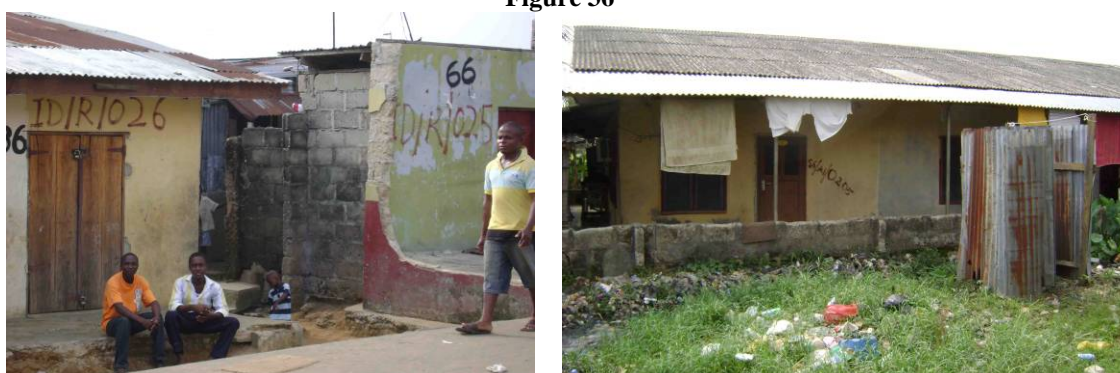
Houses in Abonnema Wharf Waterfront demarcated for demolition
