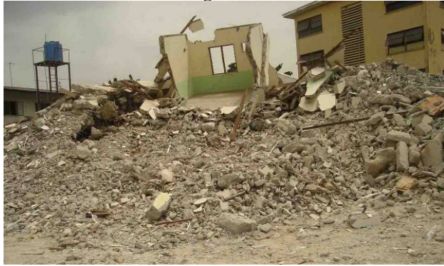
Half demolished legal buildings on Abonnema Wharf Road, during demolitions 10-13 February 2009 © SERAC
