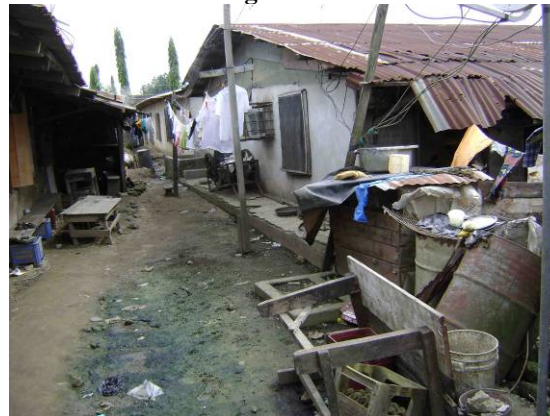
Stagnant waste water along one of the foot paths in the waterfront settlement © R. Precht
