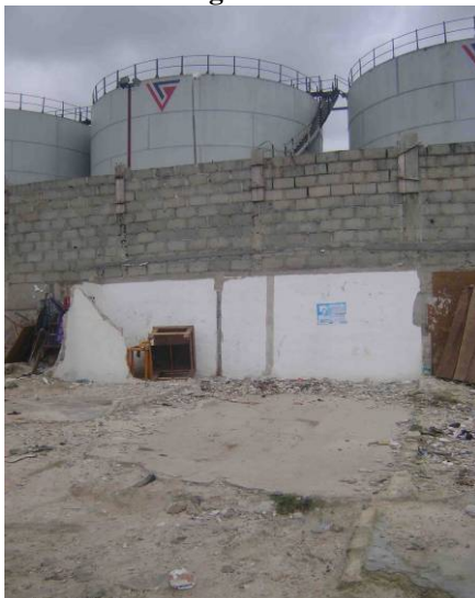
Remnants of demolished “illegal structures” used for commercial purposes along the lower part of Abonnema Wharf Road, with fuel tanks of Sigmund Nigeria Ltd. in the background © R. Precht
