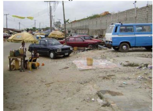
The same location as pictured left after the rubble has been removed. Only foundations and floors are left, in March 2009 © R. Precht
